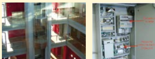
Frequency inverter for 3 phase AC motor (lift-elevator)
